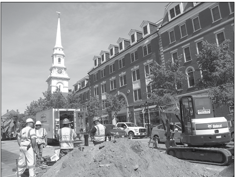
The installation of new gas lines under Congress Street has been proceeding as smoothly as could be hoped, considering that utility workers are performing exacting tasks involving a highly-flammable gas capable of producing huge explosions, all amid heavy pedestrian and automotive traffic.
